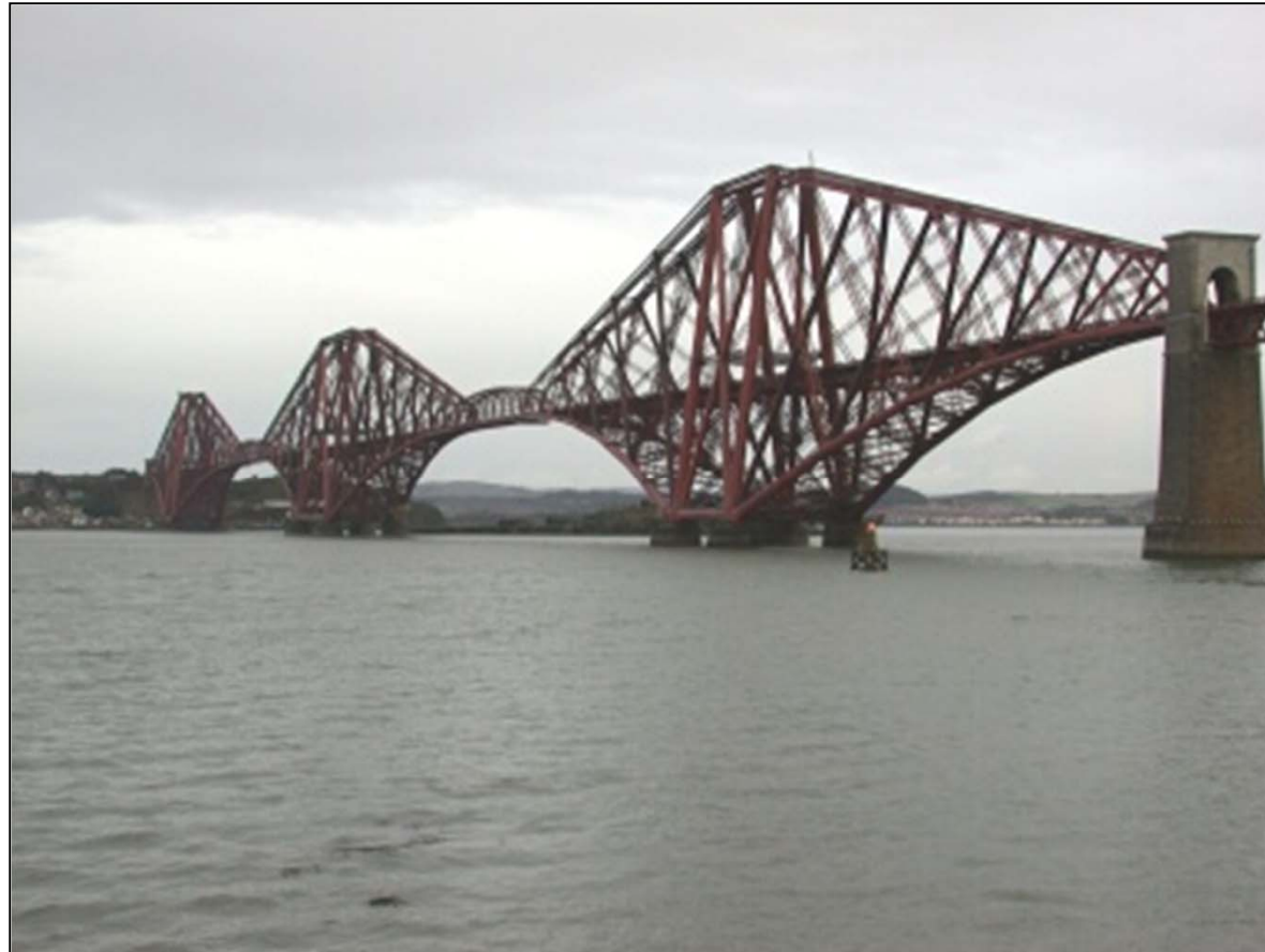
Forth Rail Bridge
